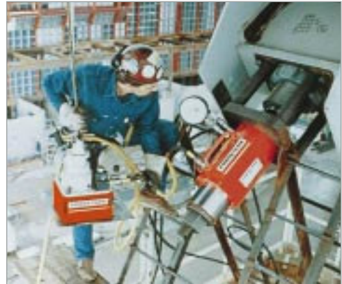
PA554 pump and RH2008 Center Hole cylinder used to tension cables.
